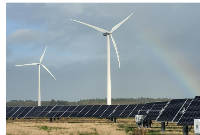
▲ Power generation facility in Holmen, Denmark, developed by EE
