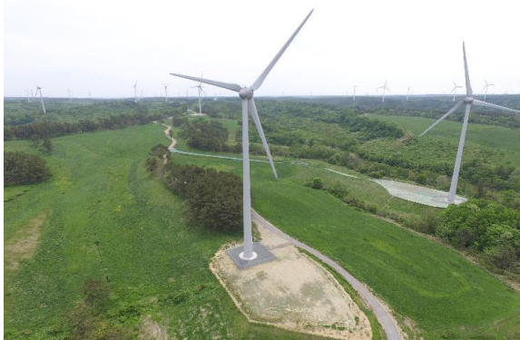
“Yokohama-machi Hibaritaira Wind Power Plant” (Aomori Pref.)
