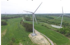
"Yokohama-machi Hibaritaira Wind Power Plant" (Aomori Pref.)
