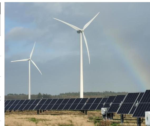
▲ Power generation facility in Sluseholmen, Denmark, developed by European Energy
