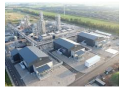
📷 1 The world's first e-methanol production plant
