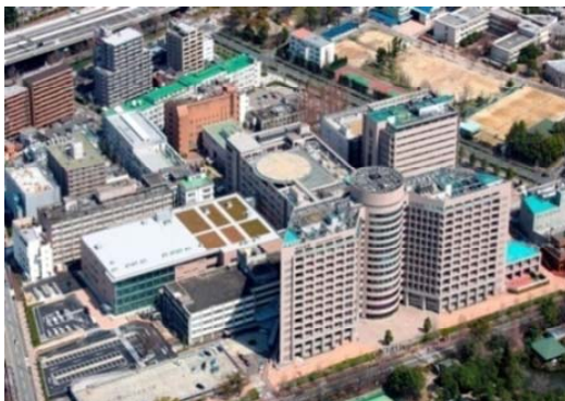
Nagoya University Hospital has introduced our ESCO in April 2010. This ESCO is expected to achieve energy saving by 20.6% and reduce CO2 emission by 21.0% (approx.7,000ton).
