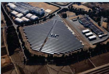
(Above) Makabe Solar Power Plant
