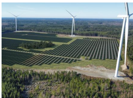
▲ Hybrid solar and wind power generation facility in Sweden (Skåramåla)
