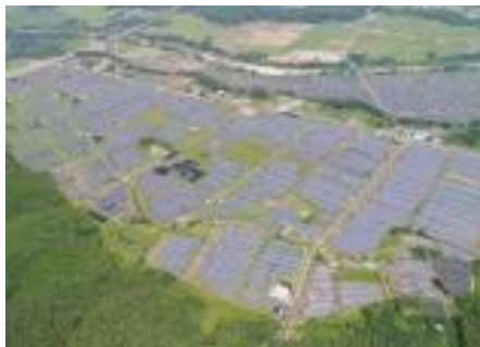
▲ Mega solar power plant in Yatsuda District of Namie Town (Fukushima Prefecture)
