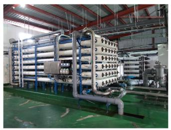
Hitachi Aqua-Tech's RO system (similar scale system for this project)
