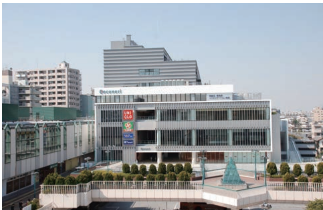
Outside view of Coconeri* 3 , one element in our social infrastructure business.
