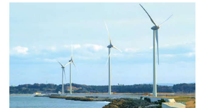
Manyo-no-Sato Wind Power Plant (Fukushima Prefecture)
