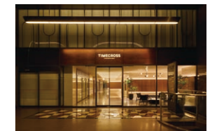
Office building after renovation
