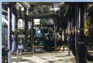
Inside of facility equipped with energy saving equipment
