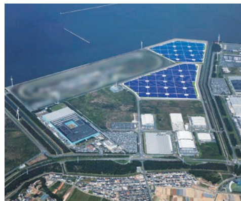
Site for construction of a megawatt-class solar power facility (Tahara City, Aichi Prefecture)
