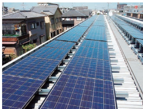
Solar power generation project using the roof of a rental apartment block
