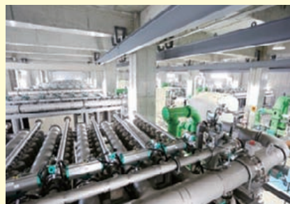
Interior of the membrane filtration plant
